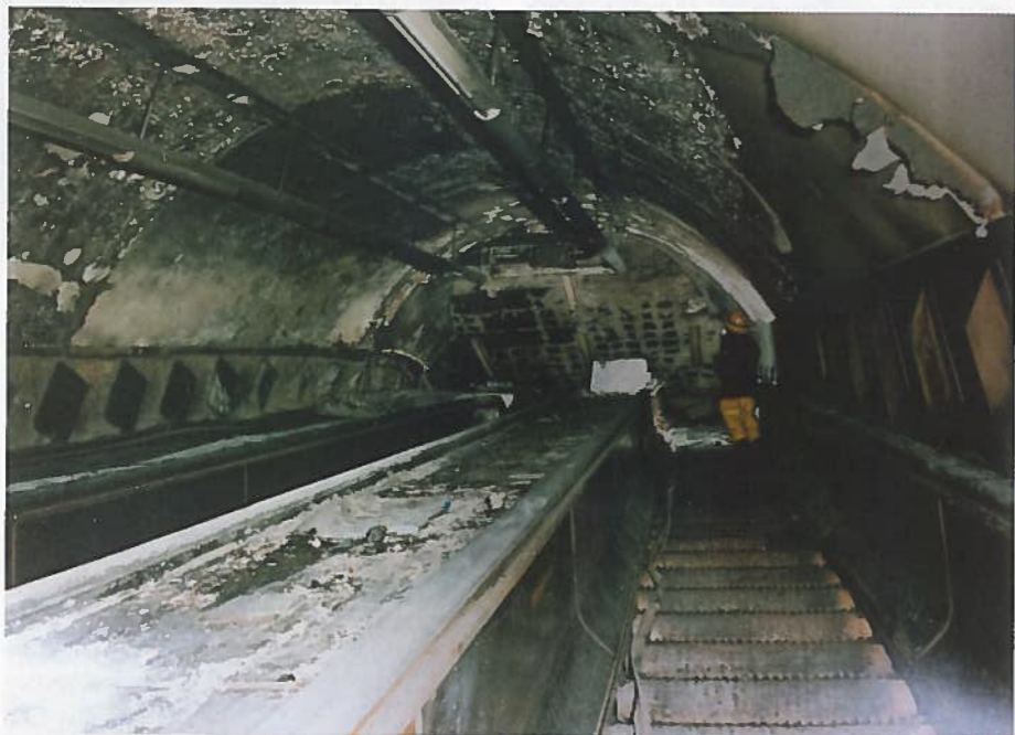
The view looking up the same shaft in November 1987 showing burn patterns. LONDON FIRE BRIGADE.
