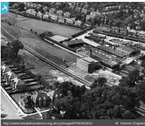
1939 doubling the track between Mill Hill East and Mill Hill the Hale. The aerial view shows John Laing's builders works and Bunns Lane running across the top. Also note the electric sub station being built alongside the track.
