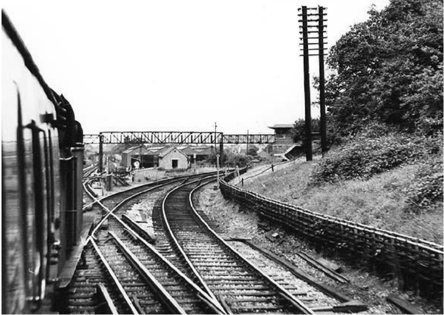
Fig 15 Park Junction at Highgate on the last day of passenger service to Alexandra Palace July 1954. Note the conductor rails in place on the south bound road, and the tube depot in the background.
